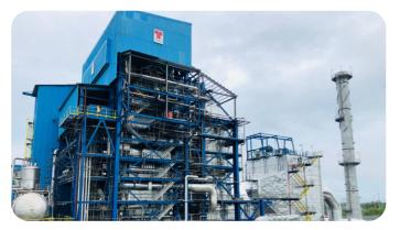
40 MW Boiler Turbine Generator (BTG) supplying steam and power to the sugar and refinery factory Source: <u>Thermax Global</u>
